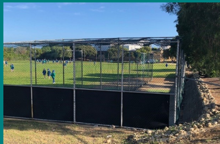
ALCOA grant—retaining wall.
