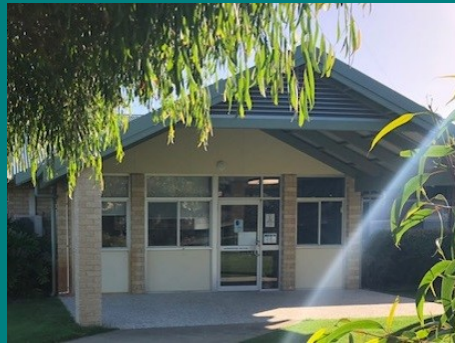
Building improvement entrance
